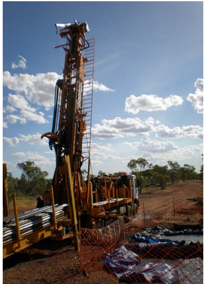
Diamond Core Drilling
