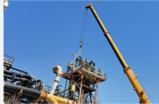
Cyclone cluster pump & pipe removal
