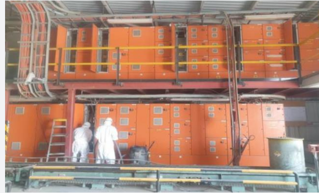
Cleaning of motor control centre (MCC) and precipitation bund
