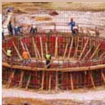
In Construction Kayelekera
